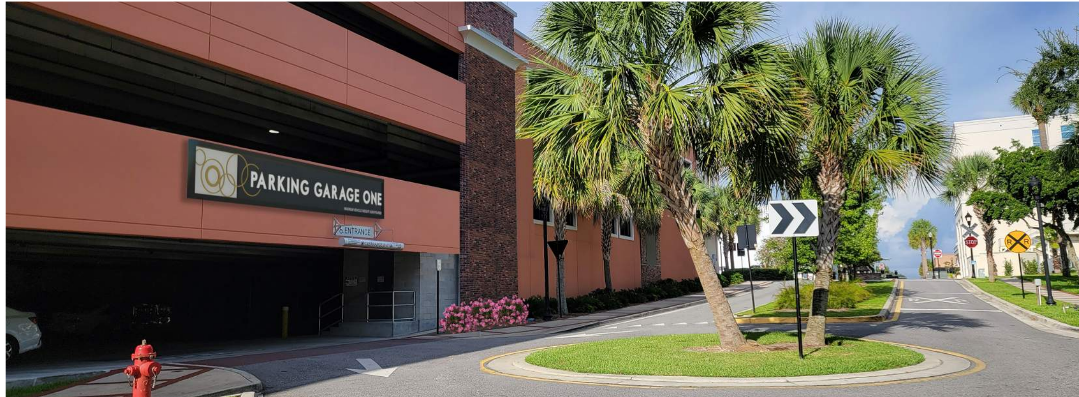
LOCATION B - VIEW 1: WEST BROADWAY STREET:
